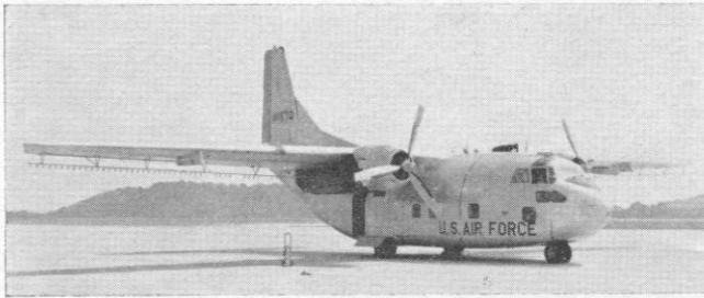
LEFT: The C-123 Provider has been given a new lease of life by the requirements of counter-insurgency forces. This C-123B-FA, 54-570, is fitted with underwing spray booms, as supplied to the 315th TCW in Viet Nam for defoliating jungle. RIGHT: Another veteran brought back into service is the A-1E Skyraider (52-132683 illustrated) which equips the 603rd and 604th Fighter Squadrons in the Air Commando Wing
